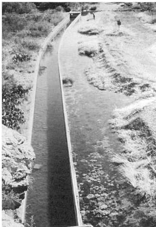
Figure 2. The Phantom Lake Spring irrigation canal and endangered fish refuge in November 1993. This view is from just above the spring outflow looking toward the Cipoletti weir that controls the exit of water from the refuge.
